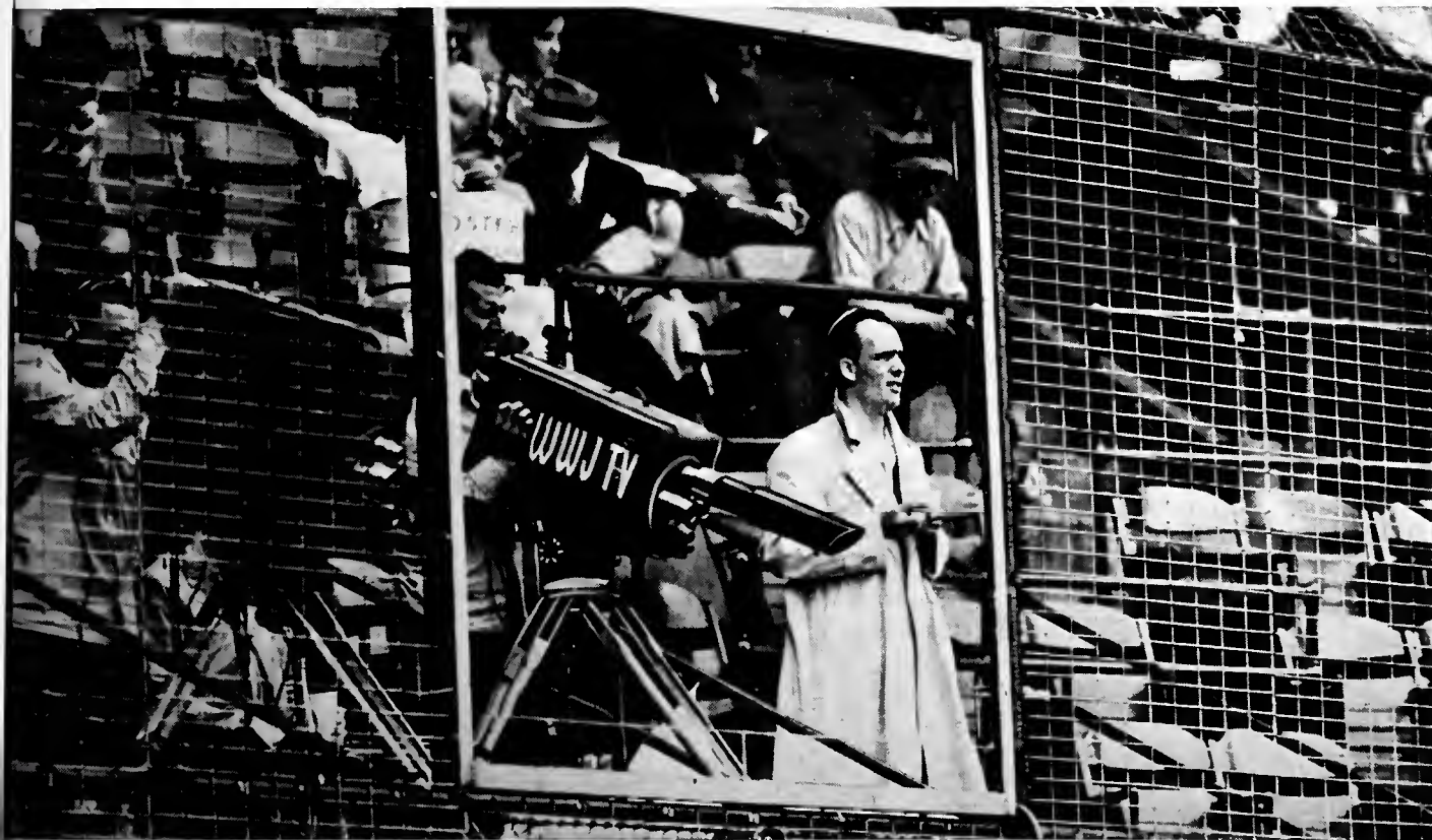
WWJ-TV's cameras are set up in the lower stands with a shatterproof glass window to shoot through. Home games
